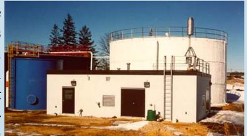
For smaller systems, covered steel or concrete tanks are used instead of lined lagoons as shown in another example. These compact systems can be built with reactor sizes up to 2.0 MG. The system above did not waste any sludge from the process in the first seven (7) years of operation, saving a considerable amount time, hauling cost, and disposal fees.
